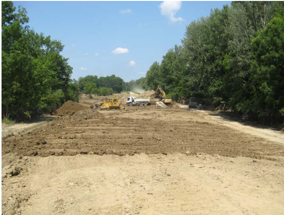
Figure 18 - Reconstruction of the Drina levee near Bijeljina
