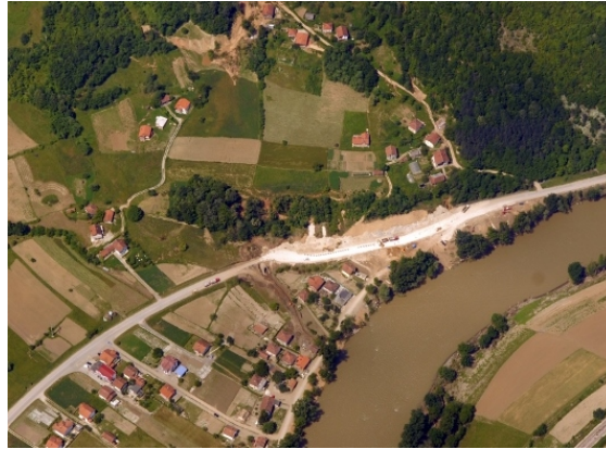
Figure 4 - Kosova village Landslide on M17 road
