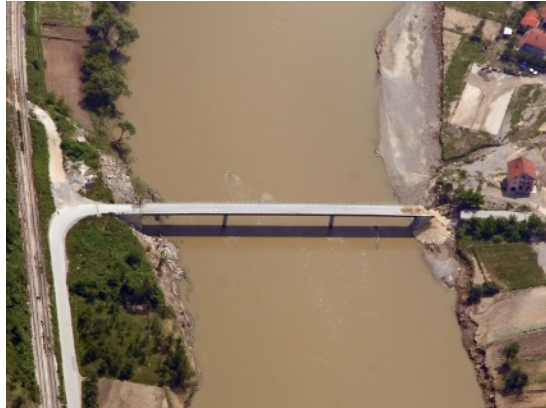
Figure 11 - Dobož bridge abutment destroyed
