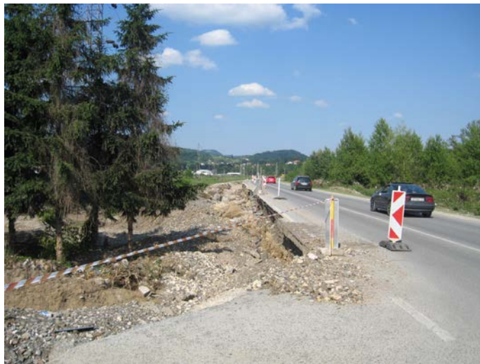
Figure 17 - Road also acting as a dyke at Dobož damaged by overflowing water.
