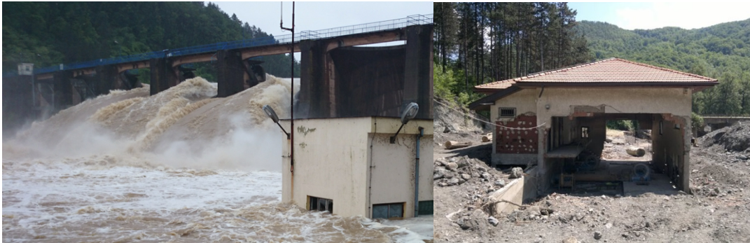
Figure 1 - Overflow at SHPP 'Modrac' (left) and destroyed SHPP near Zenica (right)
