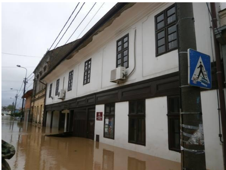
Figure 1-33. Flood Damage in Obrenovac:
