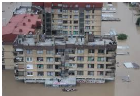
Flooded apartment blocks
