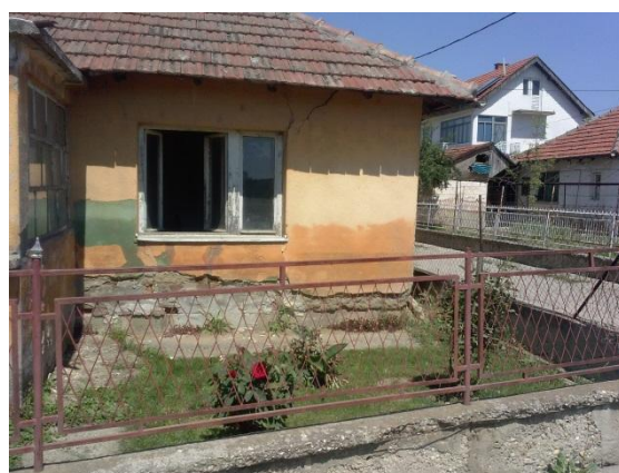
Smed. Palanka, after the flood water receded
