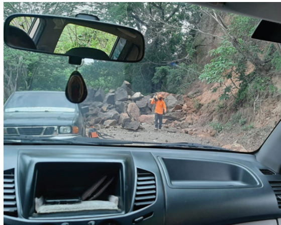
Image 8: Destroyed access to the community, road from Yayantique to Yucuaiquín.
