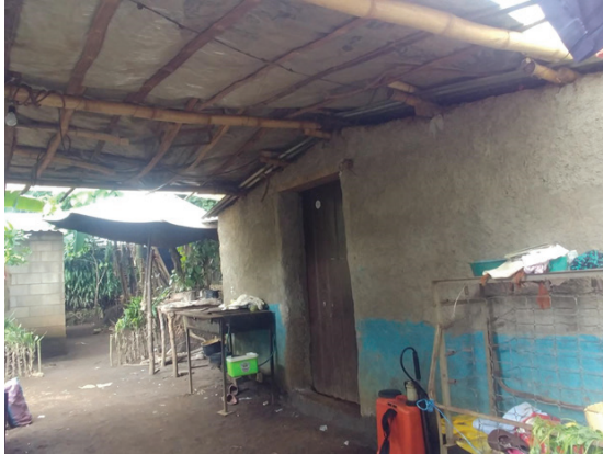
Image 1: Roof made of plastic bags on an adobe brick structure, in Cusamaluco, Nahuizalco, Sonsonate.
