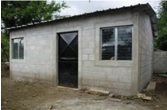
Concrete block walls with reinforced concrete columns
