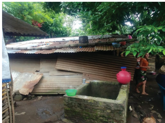
Image 9: Conditions of houses made of metal sheets, Nahuizalco, Sonsonate.
