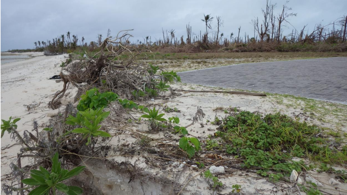
Photo 22. High exposure of Farquhar’s airstrip to cyclonic waves at its southern end
