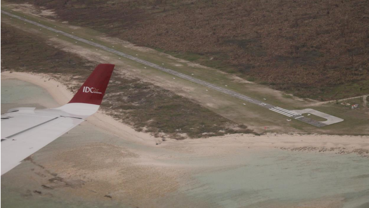
Photos 21. High exposure of Farquhar’s airstrip to cyclonic waves at its northern end
