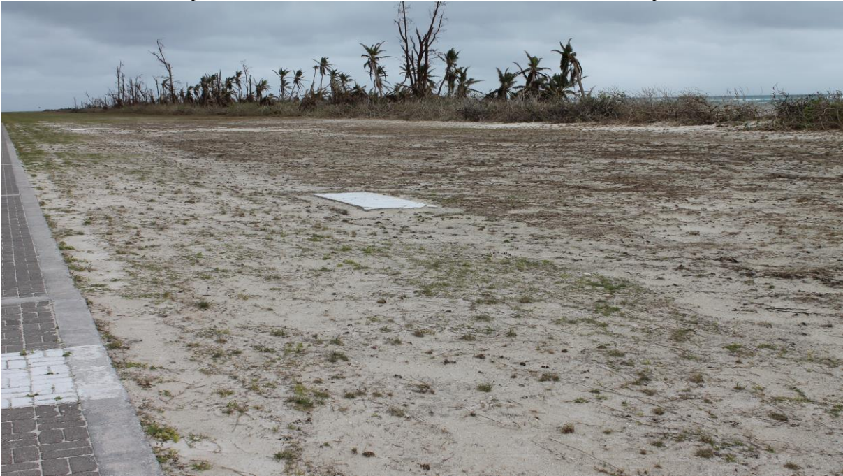
Photo 23. Extended deposition of sand and coral debris in the axis of the airstrip
